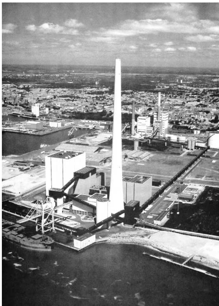
FIGURE 1.1 A power station in Esbjerg, Denmark.
